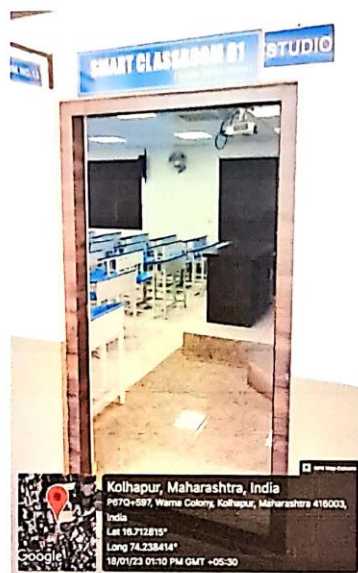
B. Renovation of class rooms Renovation of class room-1(13): Smart class room-1
