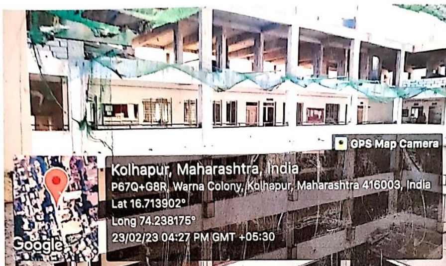
A. Construction Floor view of Physics Department
