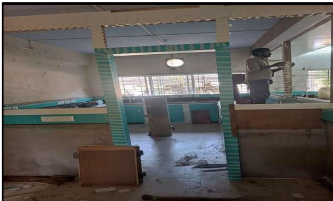
Chemistry laboratory: Renovation
