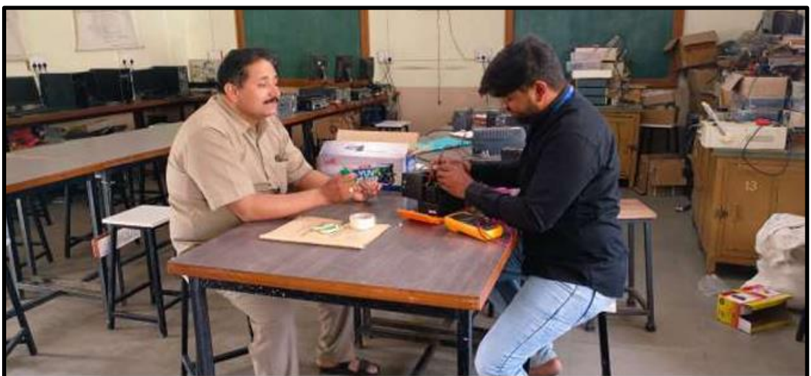
Electronics staff replacing UPS battery
