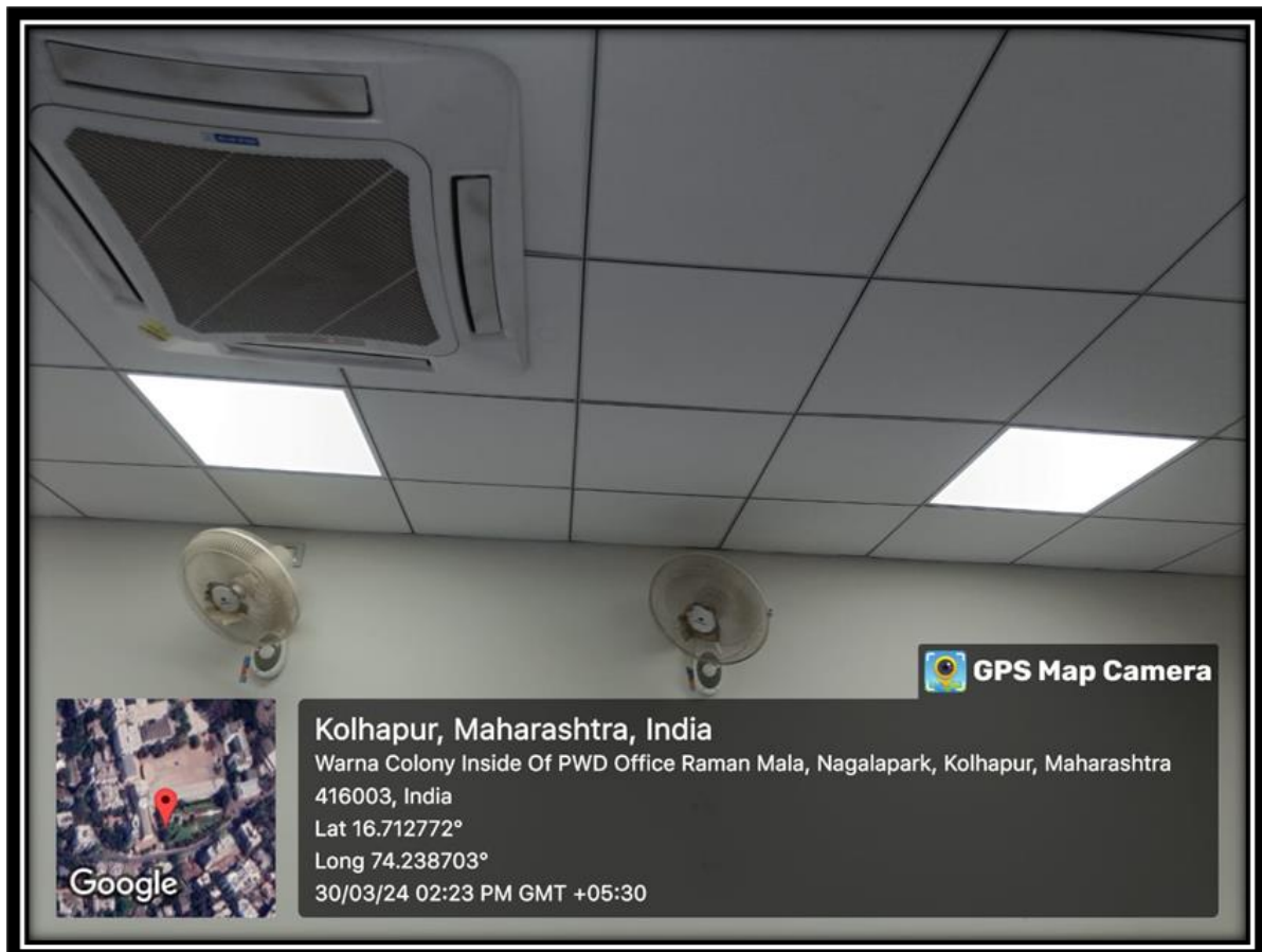
Picture 6: LED bulbs at smart room no.19
