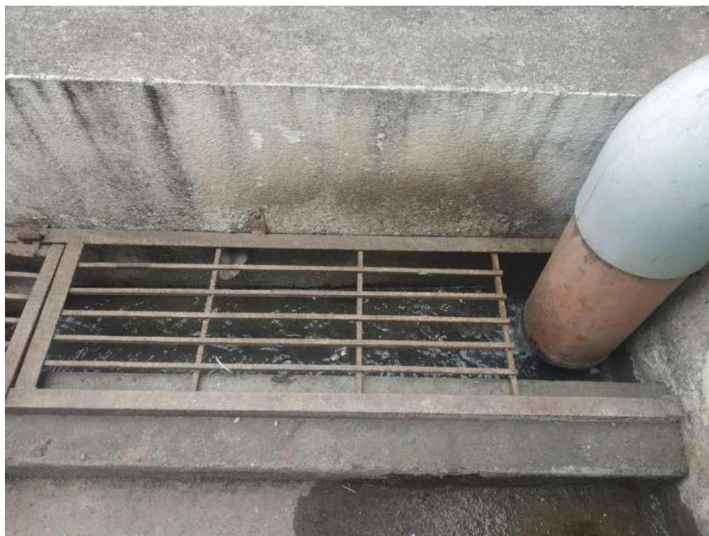
Picture1. Water from the labs is disposed in the soil under the ground
