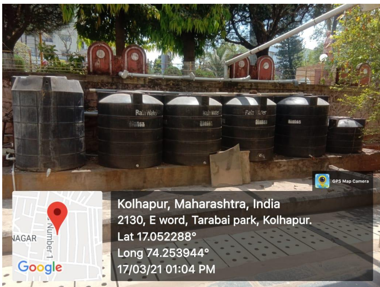
Picture: 1 Rain water collection and storage at Vivekanand Colleg
