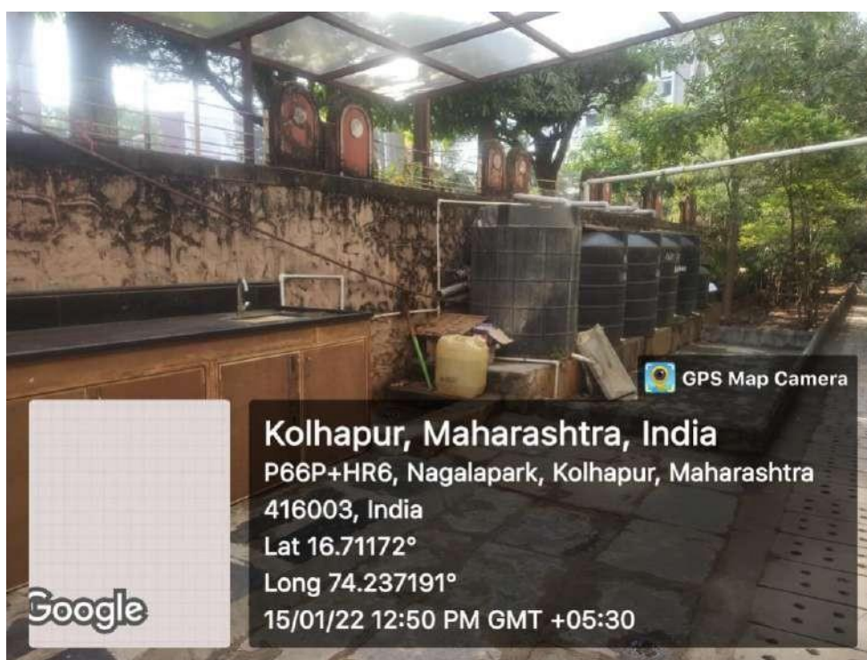
Picture 1. Rain Water is collected in 5 Syntax Tanks of around 5000 liters
