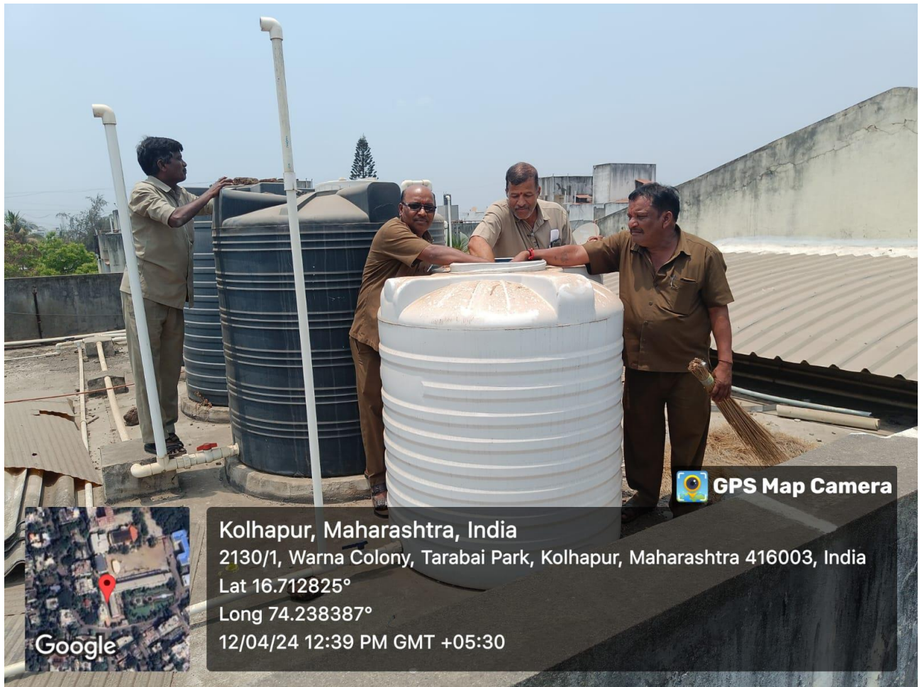
Picture1. Water tanks cleaning
