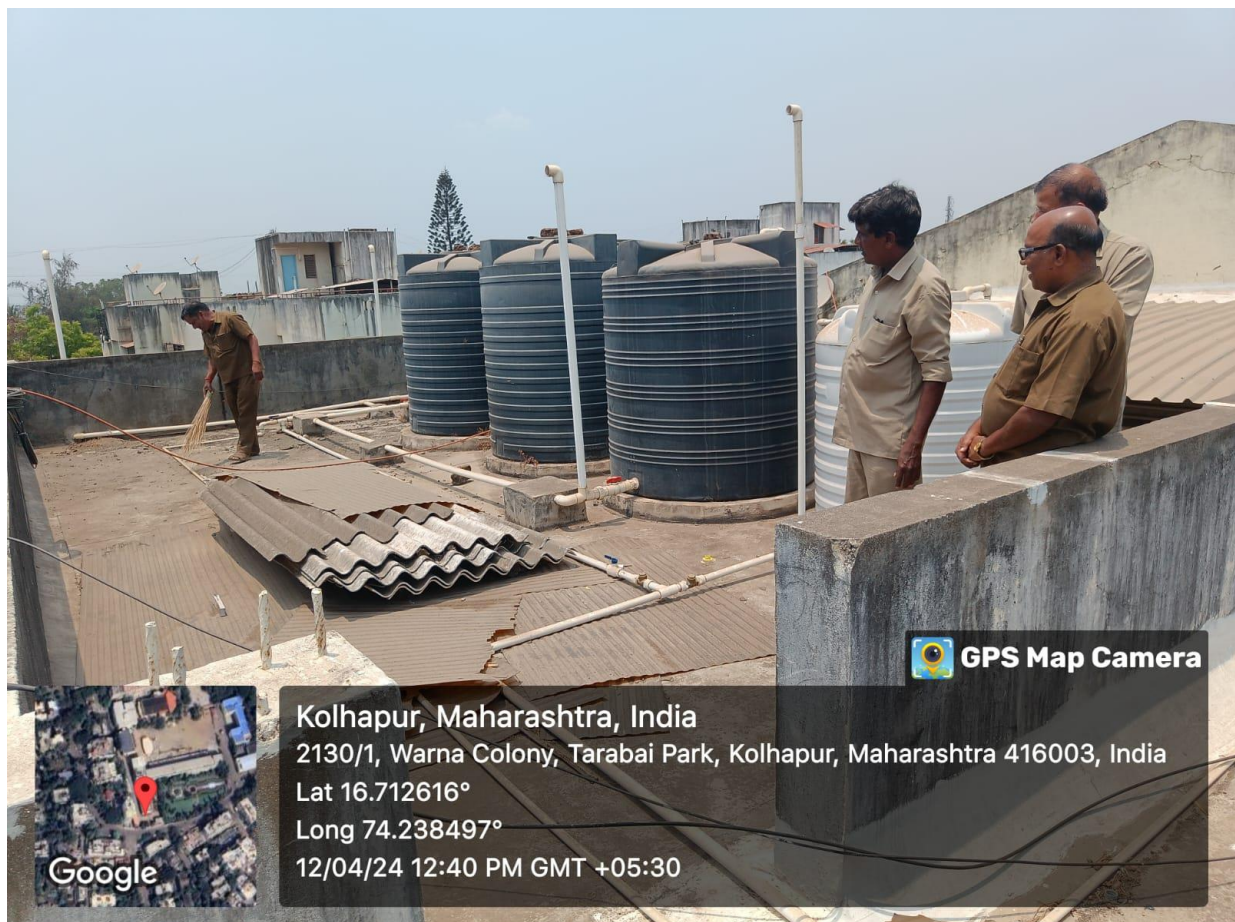
Picture2. Water tanks cleaning
