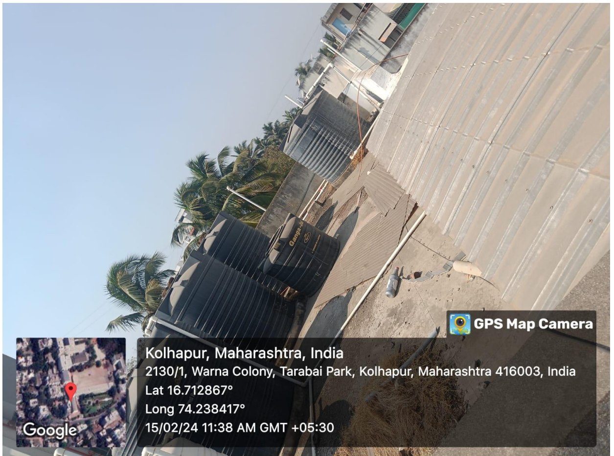
Picture 4. Water Tanks on the senior building
