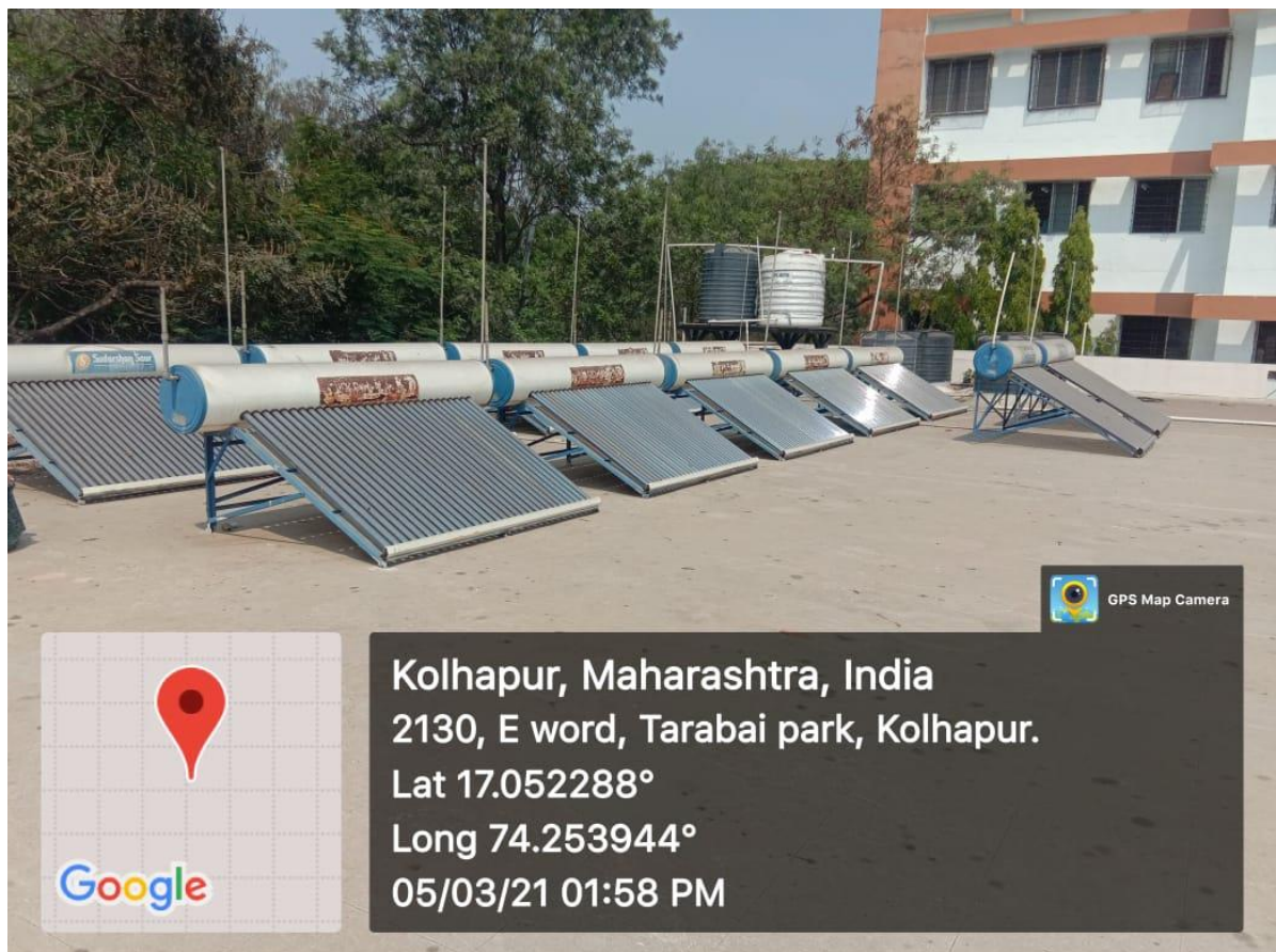
Picture 2. Water Tanks on the ladies Hostel 2
