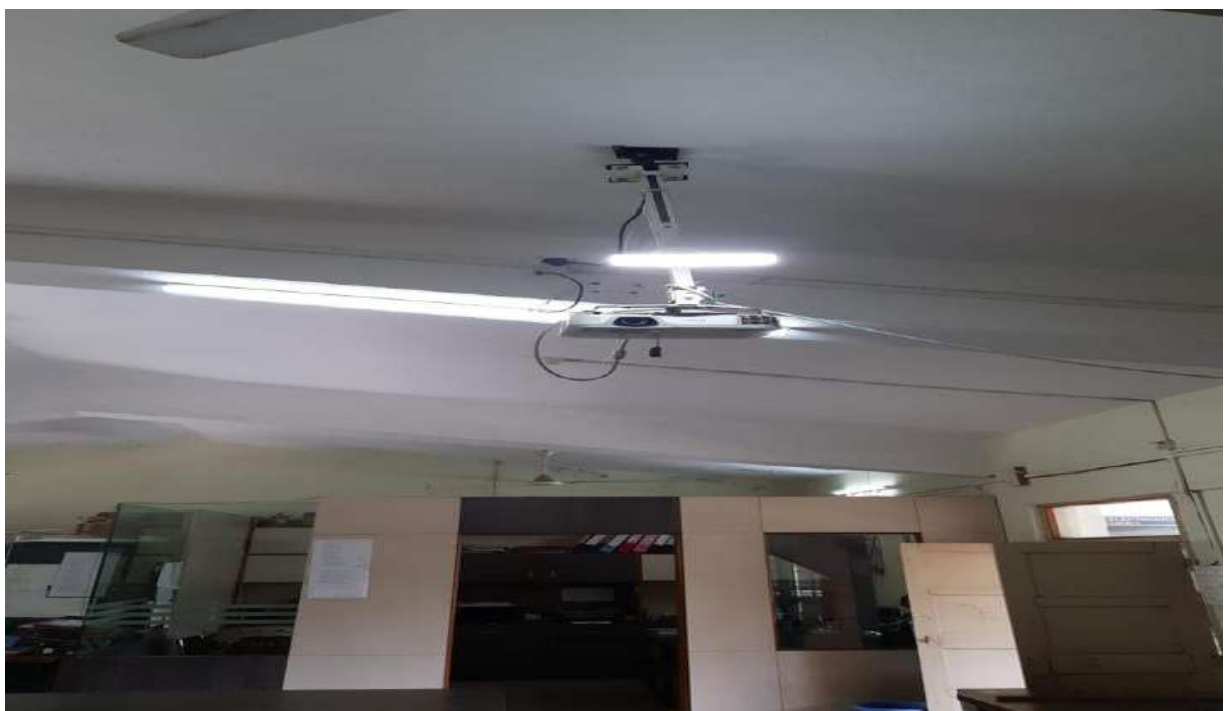
Plate No. 11 & 12: Replacement of incandescent bulbs by LED tubes.
