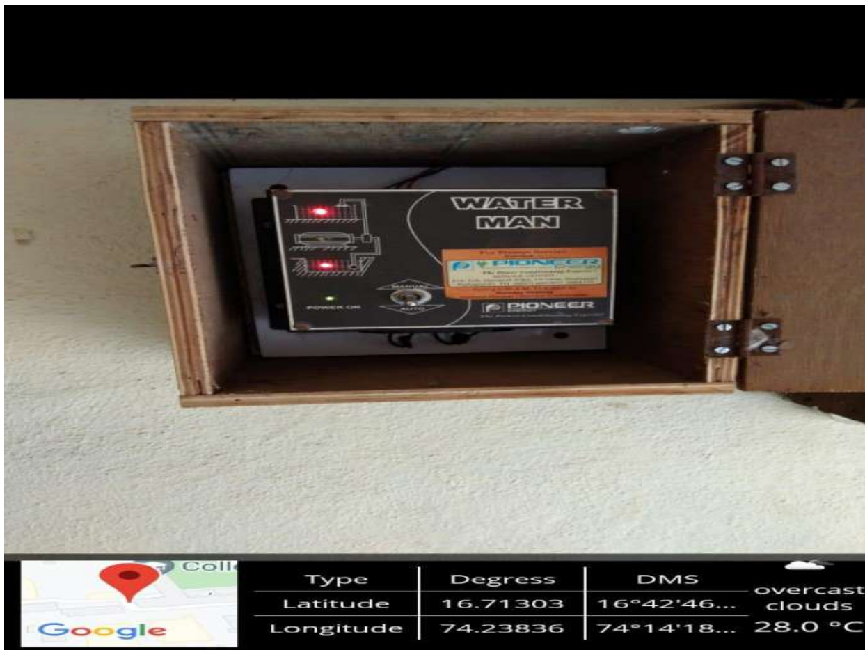
Plate No. 20: Sensor based Auto switch is used for bore well motor
