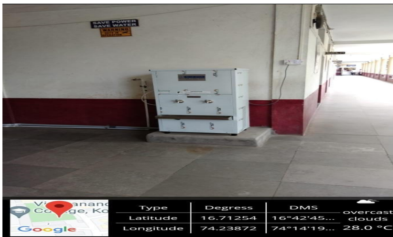
Plate No. 19: Water filter and Cooler at Vivekanand College, Kolhapur.
