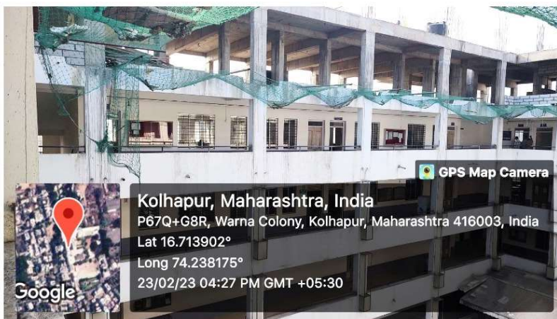
A. Construction Floor view of Physics Department
