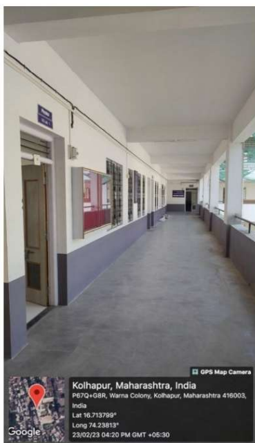
A. Construction Department: Physics Passage= (size 2.75 x 33.75 m=92.81 m 2 )
