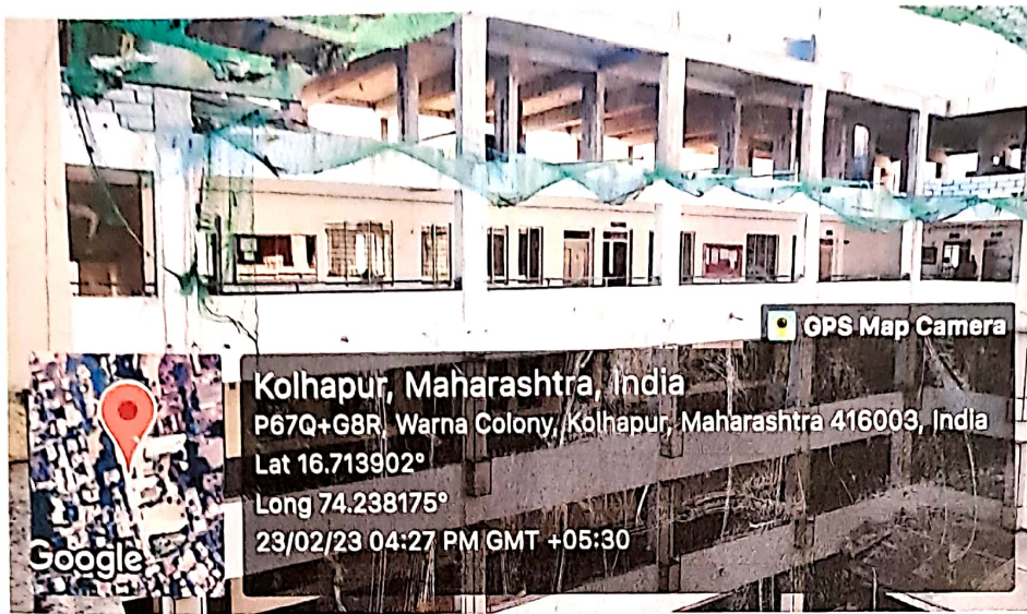
A. Construction Floor view of Physics Department
