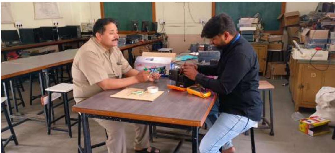
Electronics staff replacing UPS battery
