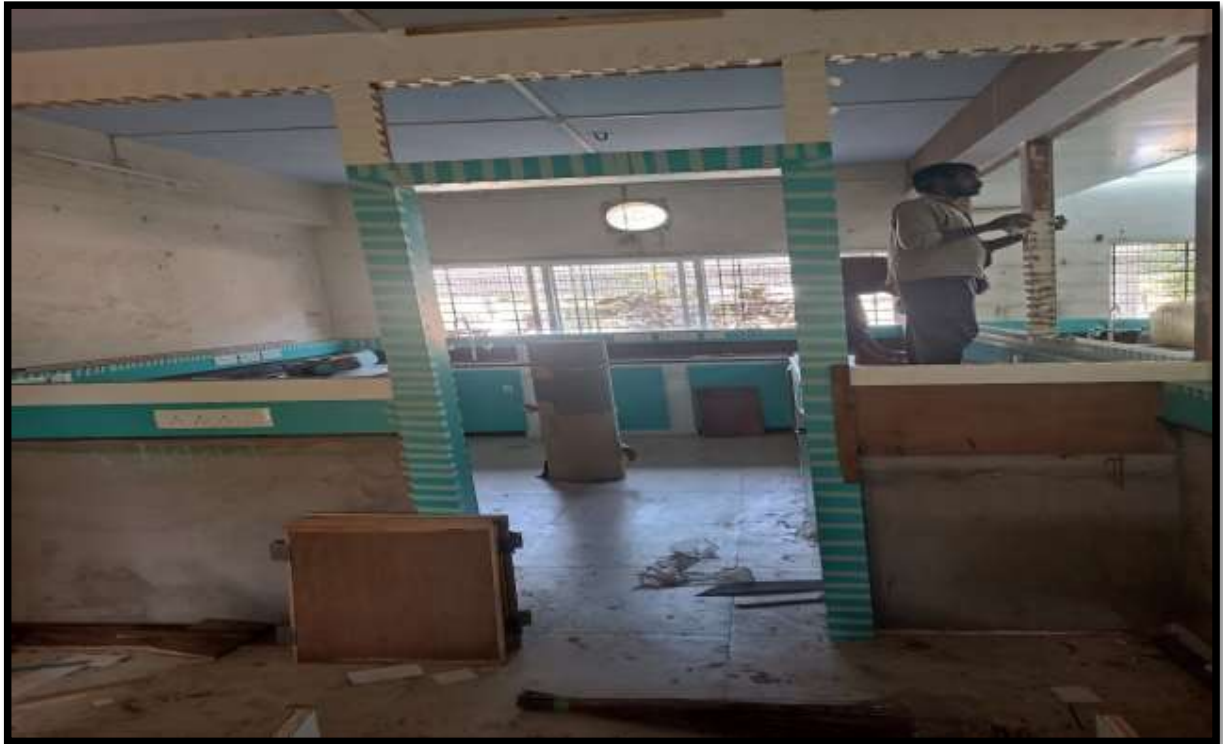
Chemistry laboratory: Renovation
